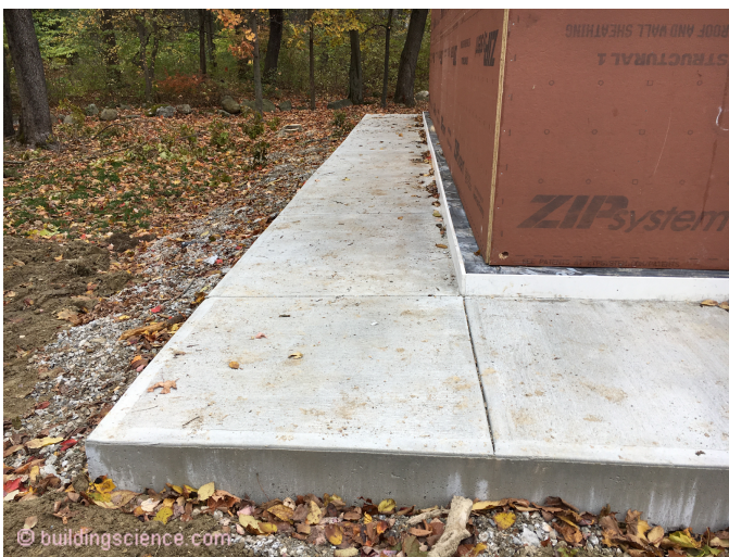
Photograph 8: Concrete Skirt – Protecting rigid horizontal insulation
