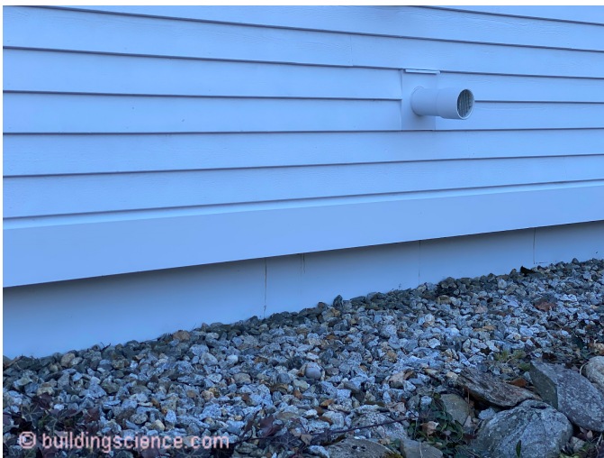
Photograph 4: Current Condition - Looking almost brand new.
