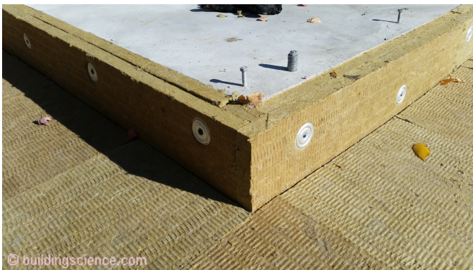
Photograph 7: Shallow Frost Protected Foundation – Rigid horizontal insulation.
