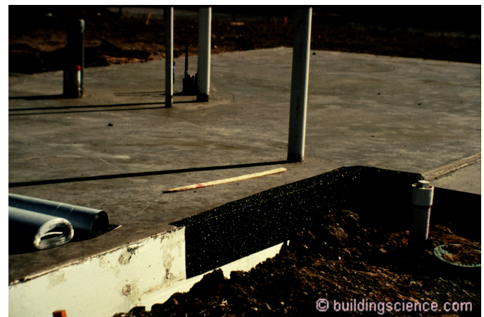
Photograph 2: Fully Adhered Membrane - “Roofing” strip used to protect slab edge insulation.
