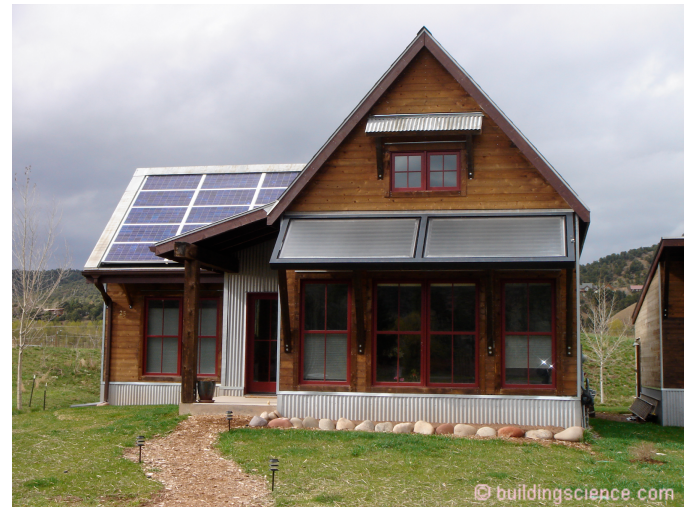
Photograph 5: Carbondale, CO - Exterior foundation insulation is protected by rigid metal sheeting.
